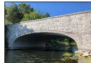
Figure 5: Three-sided Box Bridge
